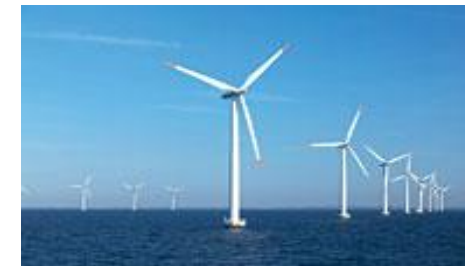
Off shore wind turbines
